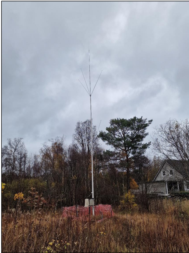
Comrod antenna for 1314 East of Transmitter House at LKB LLE.
