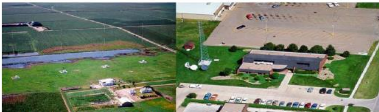
Transmitter Site Holdrege, Ne.
