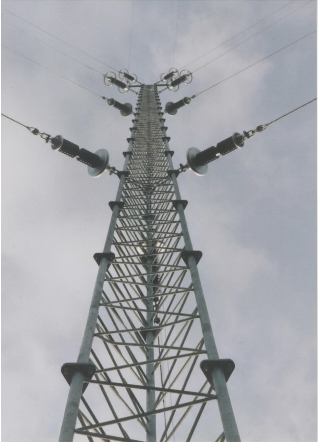
ICB 549 kHz transmitting mast, Photo: Engineer Peter.
