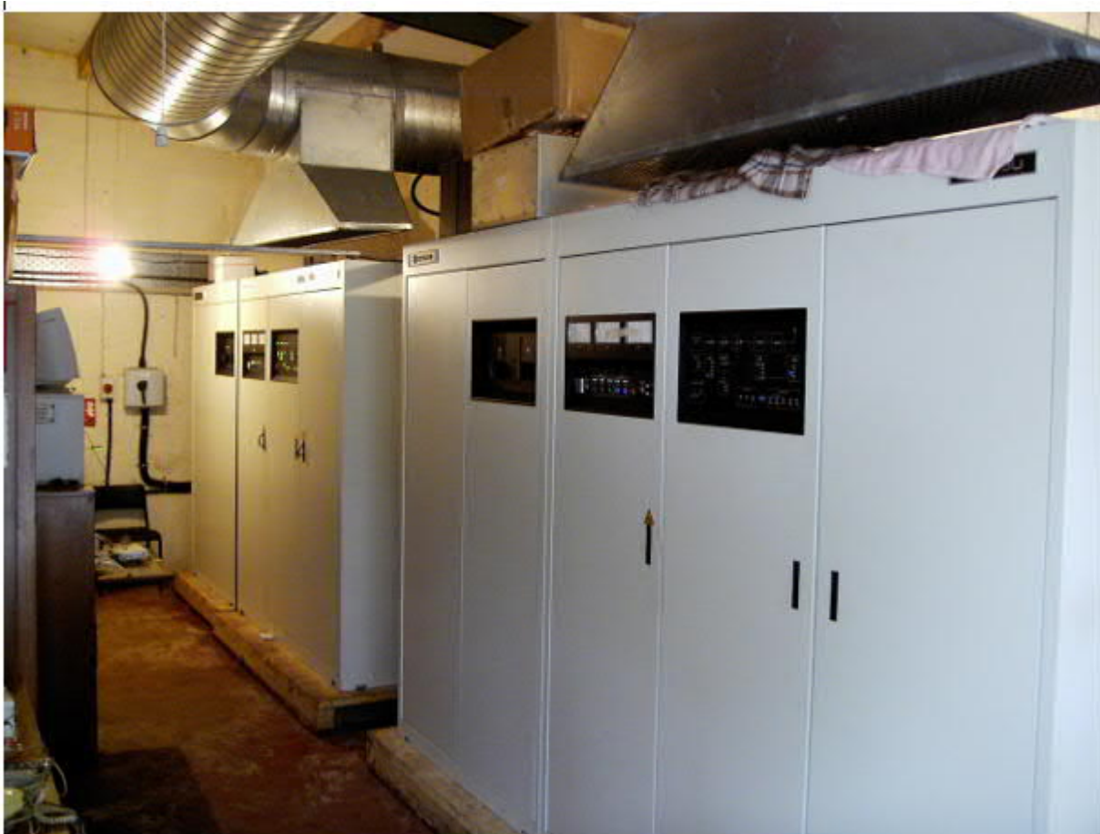
549 kHz transmitters, two Harris DX25, and one Transradio 50 kW. Photo: Engineer Peter
