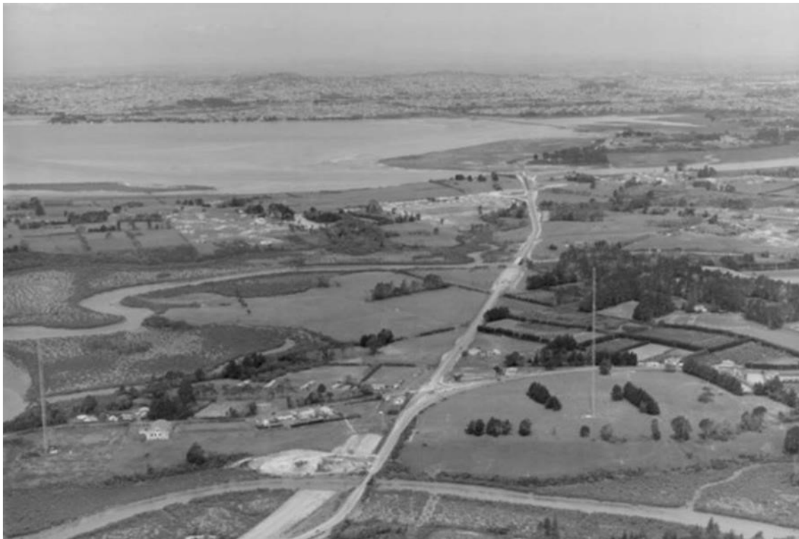
Picture: Auckland Henderson sites 1955 taken by Whites aviation with Auckland city in background
