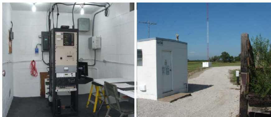
Transmitter Equip. Cozad, Ne
