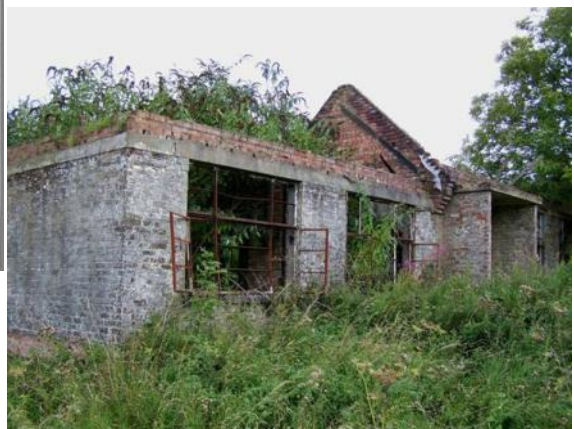
A.E.i.C and Clerical Staff offices - the roof collapsed some years ago following heavy snow.
