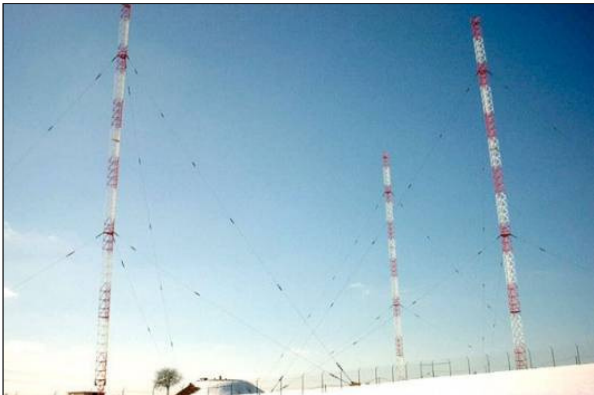
The medium wave antenna at Marnach, Luxembourg
