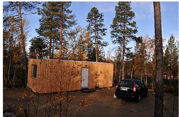
The cabin has a new wooden siding.
