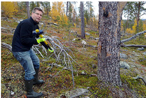
Jim hammering a grounding rod at the end of the new 160-degree antenna.
